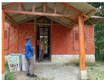
Figure 4.5 Supporting Facilities, complete with toilets, kitchens and lodging in the forest
